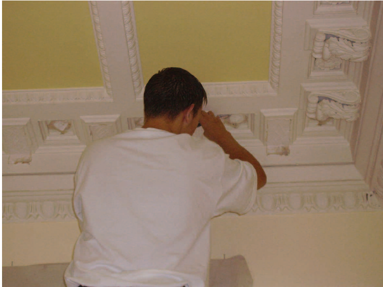
Paul Malyon removing enrichments. The paint was removed in our workshop, then modelled and reset.
