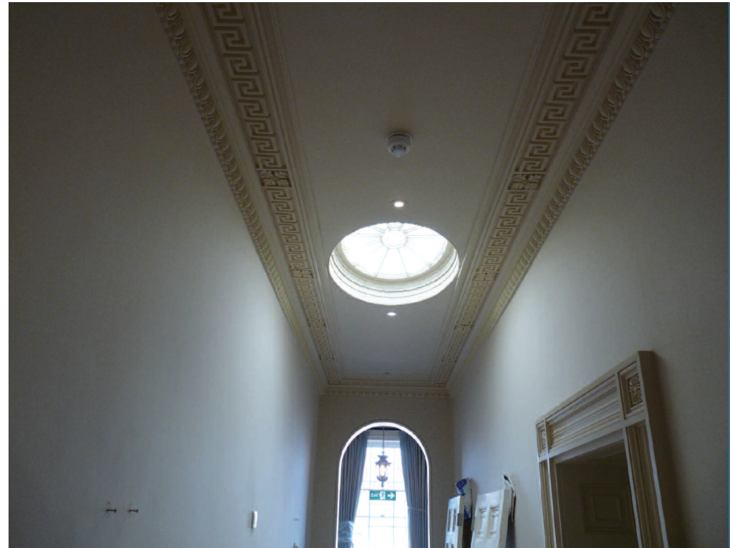
1st floor east corridor cornice and circular skylight restored.
