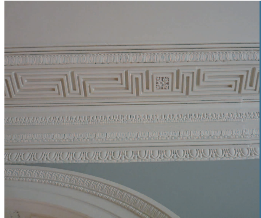
New enrichments bedded in complete new section.
