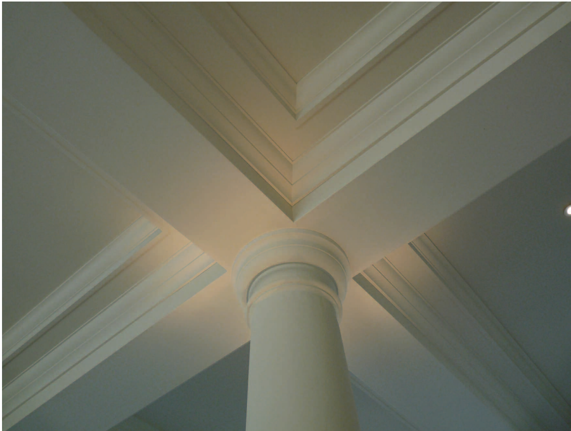
GRG Column and beam casings completed and decorated.
