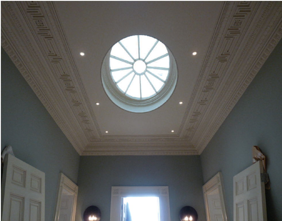
1st floor west corridor cornice and elliptical skylight restored.
