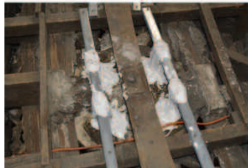
Reinforced walkway and new wadding for enrichment fixings.
