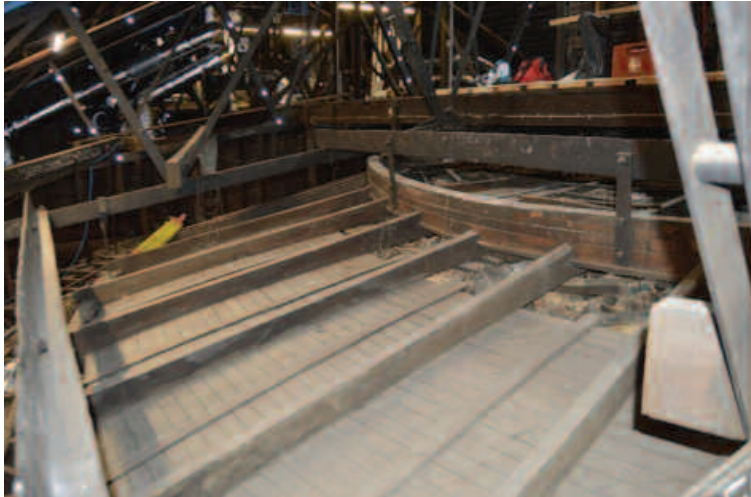
Walkway prior to reinforcement.
