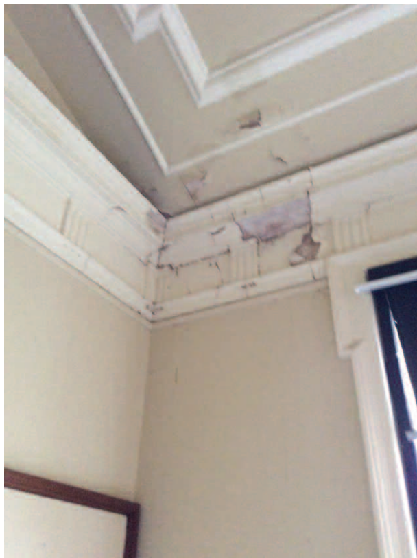
Damage to existing ceilings.
