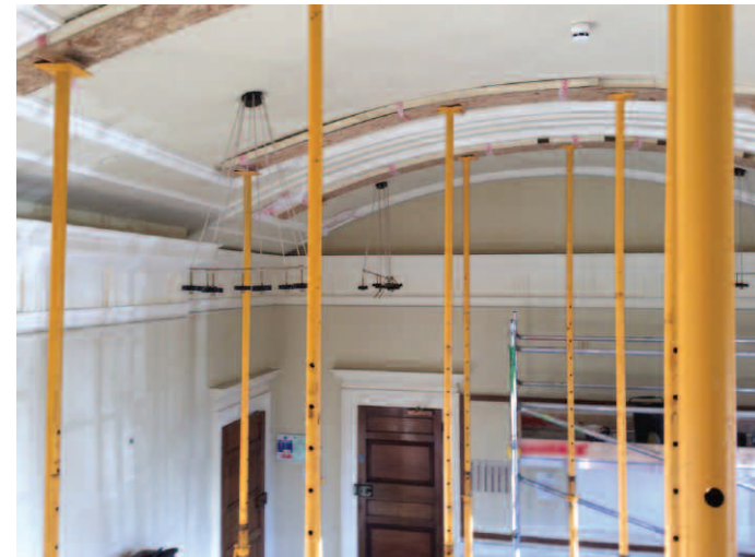
Original ceiling supported to prevent collapse.
