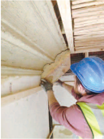
Running up core for a cornice.
