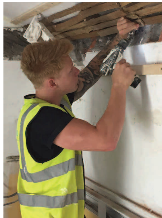
Our apprentice Jake fixing wooden laths.
