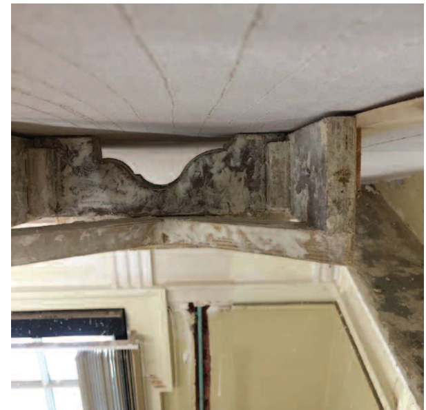
Shaun Chamberlain running the core for rib moulding on a semi-circular barrel vaulted ceiling.
