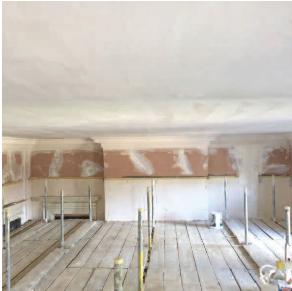
Lath and three coat sand and lime ceiling, cornice and ceiling moulds run insitu.
