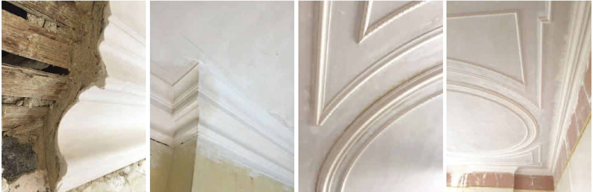
Lath and three coat sand and lime ceiling, cornice and ceiling moulds run insitu.
