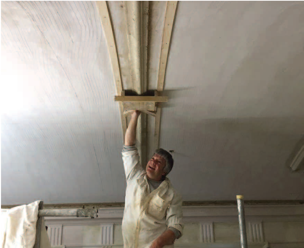
Shaun Chamberlain running the core for rib moulding on a semi-circular barrel vaulted ceiling.
