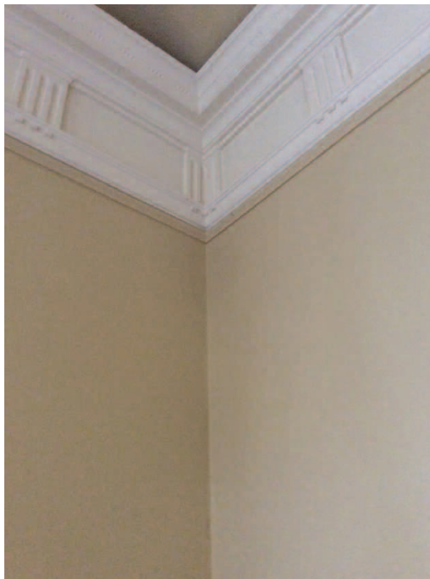
Completed cornice reinstated.
