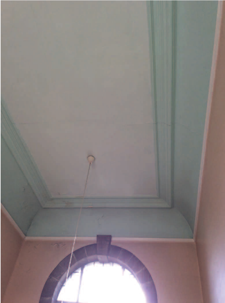
First floor original cornice to be replaced.
