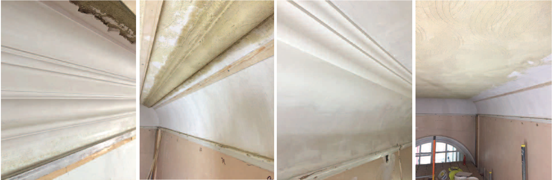
Corridor ceiling lath three coat sand lime and large cove run insitu.
